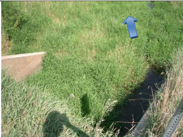
Flow through the right barrel.
