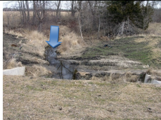
The deposition upstream is asymmetric. The picture shows that culvert was recently cleaned.
