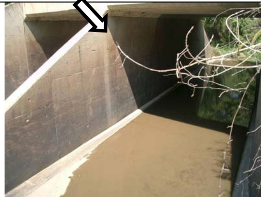
The barrel is clean. Water mark (white arrow) shows high flow condition
