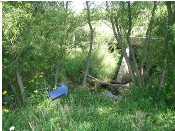
Three-barrel culvert with two barrels blocked by debris and sediment.
