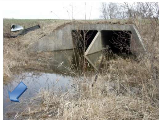
View of culvert exit
