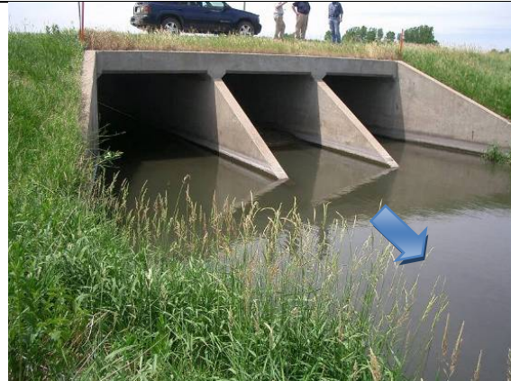
Culvert outlet clean. Sedimentation is in the central barrel
