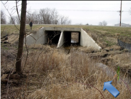
Upstream culvert side
